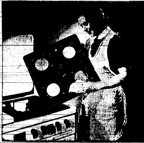
Burners of modern gas ranges are of the non-clog type and require little cleaning, but if the flame openings become clogged, clean with stiff brush or gently insert small wire to free obstruction.
